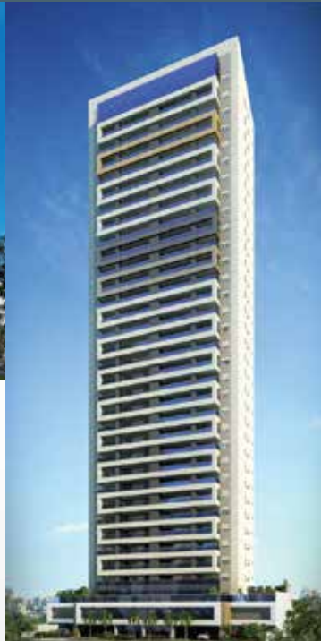
Park Line Urban House
